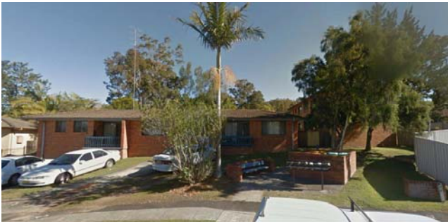
EXISTING 1 STOREY MULTI UNIT DEVELOPMENT
