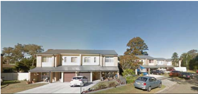
EXISTING 2 STOREY MULTI UNIT DEVELOPMENT
