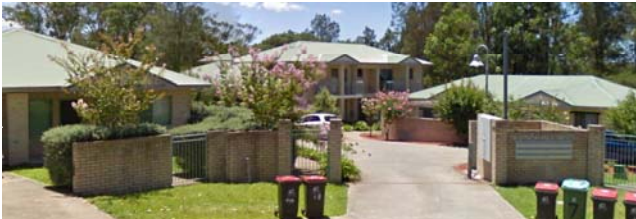
EXISTING 1 & 2 STOREY MULTI UNIT DEVELOPMENT
