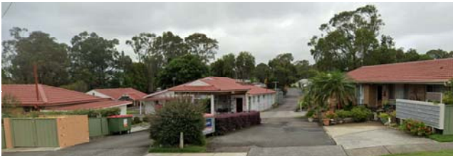
EXISTING 1 STOREY MOTEL / CARAVAN VILLAGE
