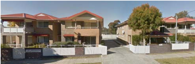
EXISTING 2 STOREY MULTI UNIT DEVELOPMENT
